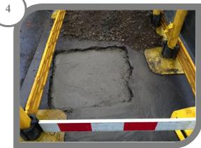
Concrete within the excavation should be reinstated to match the existing concrete thickness minimum 100mm
