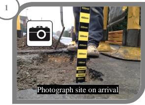
Always re-compact the sub-base Before placing any material
