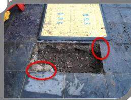
Any concrete found as a strengthening foundation must be replaced, depth to match existing minimum 100mm
