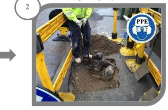
Finish concrete to the same level as the existing concrete and if it is the running surface texture it to match the existing
